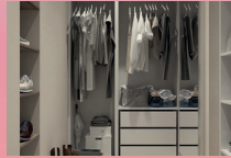
Joints around fitted wardrobes
