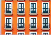
Joints around window sills, window and door frames
